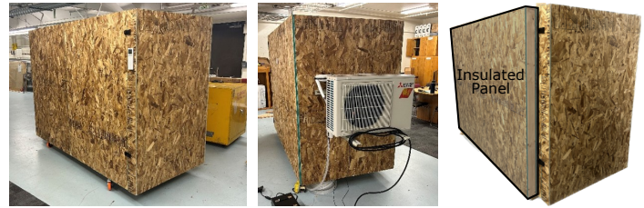
Figure 3. Testing set-up for the insulated retrofit panel using a unit cell conditioned by a heat pump
